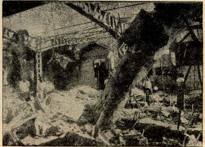
Madras Airport : Bomb blast damage
