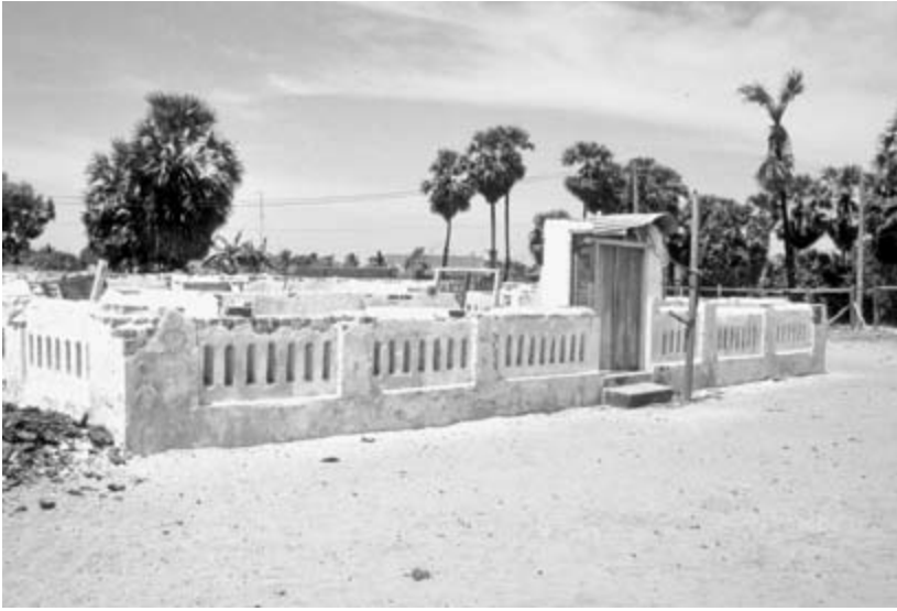
FIGURE 41. The roof and walls of this ancestral Maulana family mausoleum in Kattankudy were razed in 2004 by a Muslim fundamentalist group, although the graves themselves were not disturbed (2005).
