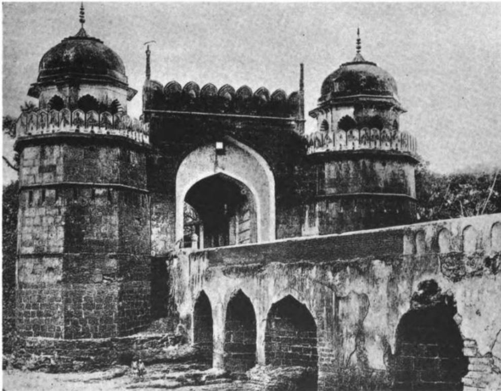
FIG. 19. BĪJĀPUR, FORTRESS GATE (AFTER REUTHER)
