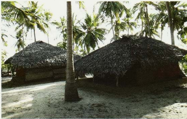
Traditional dwelling places which was constructed with Mud, Coconut Leaves at Kuṭumiyaṅ
