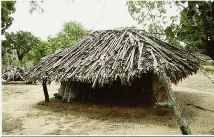
Traditional dwelling places which was constructed with Mud, Palmyra Leaves at Nelliyaṭi (Māyakkai)
