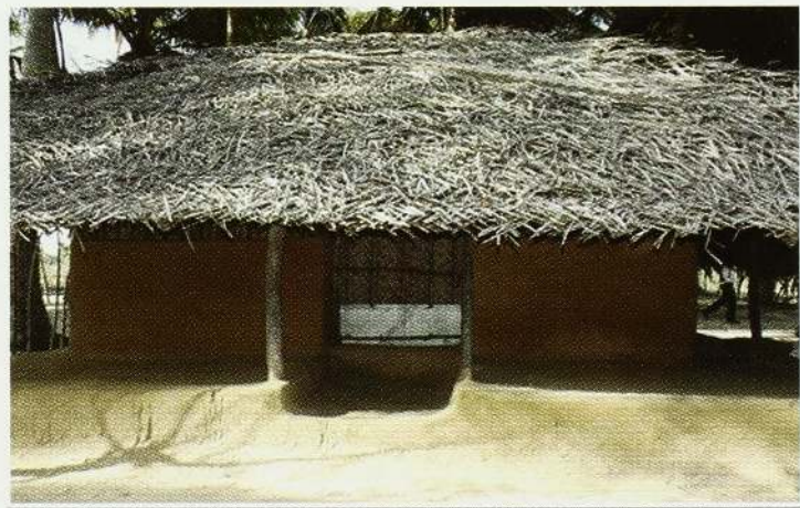
Traditional dwelling places which was constructed with Mud, Coconut Leaves at Kuṭumiyaṅ
