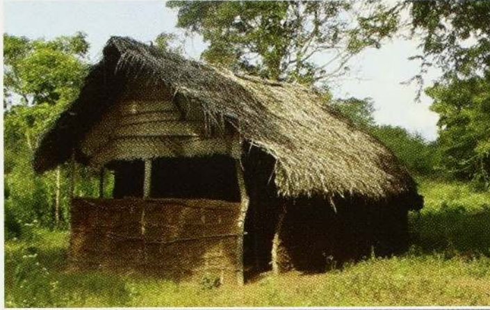
Traditional dwelling places which was constructed with Mud, Coconut Leaves at in Mullaitivu
