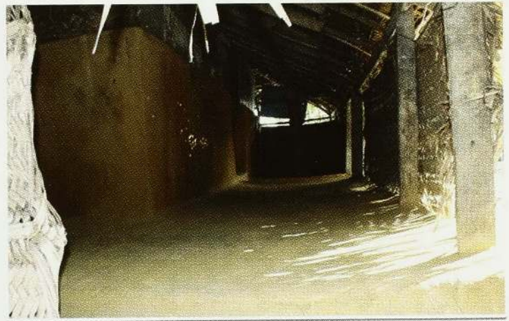
Traditional Veranda which was constructed with Mud, Coconut Leaves at Kuṭumiyan
