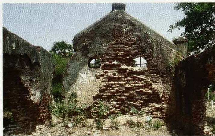
Dutch Church at Arippu in Mannār
