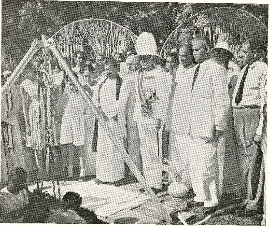
The Governor-General, Sir Oliver Goonetilleke, at the ceremony connected with the laying of the foundation stone for the Mausoleum which the Government is constructing at Horagolla to house the remains of the late Premier's body
