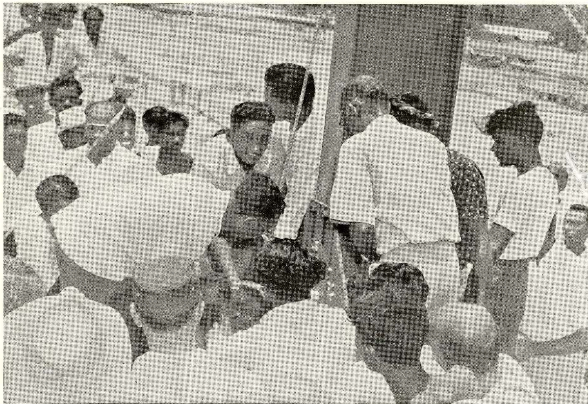
Mr. C. P. de Silva as Minister of Lands and Land Development, placing the first iron girder to construct the Sugar Factory at Gal Oya in September, 1958
