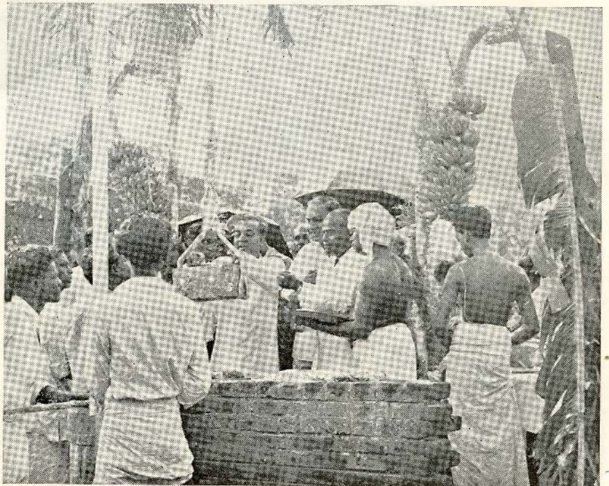
▶ Mr. Kalugalla laying the foundation stone for the new Railway Station at Jaffna
