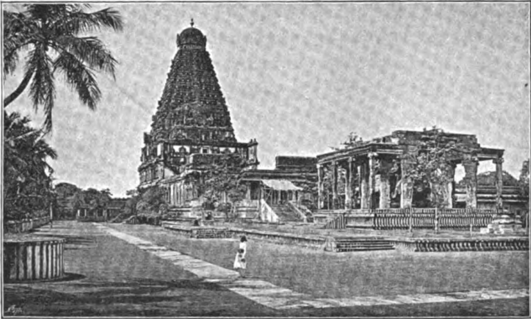
TEMPLE AT TANJORE, GENERAL VIEW.
