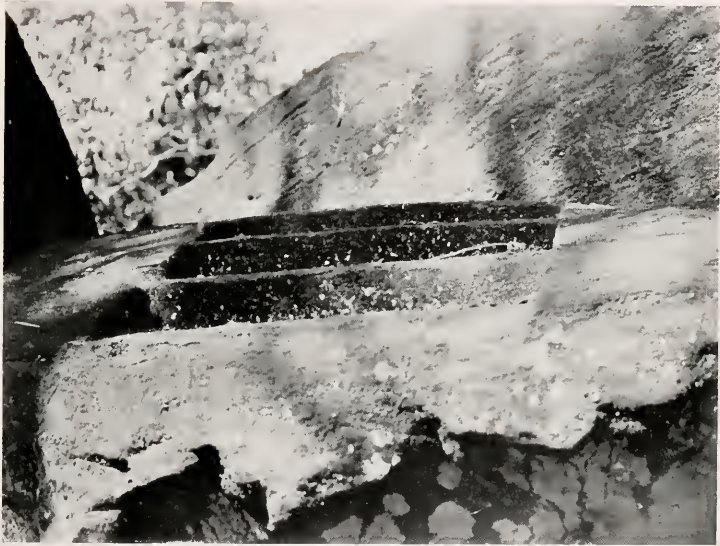
Steps cut in the rock at Bendiyalgalge
