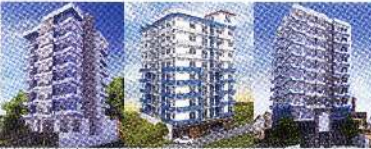
CONSTRUCTIONS OF ALL BLUE OCEAN GROUP'S LUXURY EUROPEAN STYLE APARTMENTS @ MOUNT LAVONIA, DAMBALAPITIYA, KOLLEUPITIYA & WELI LAYATTE
