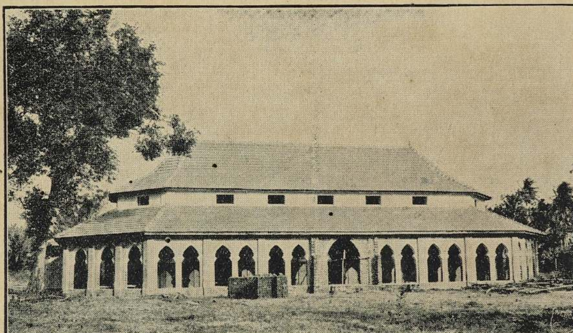
VIEW OF THE COMPLETED CENTRE BLOCK (ASSEMBLY HALL).
