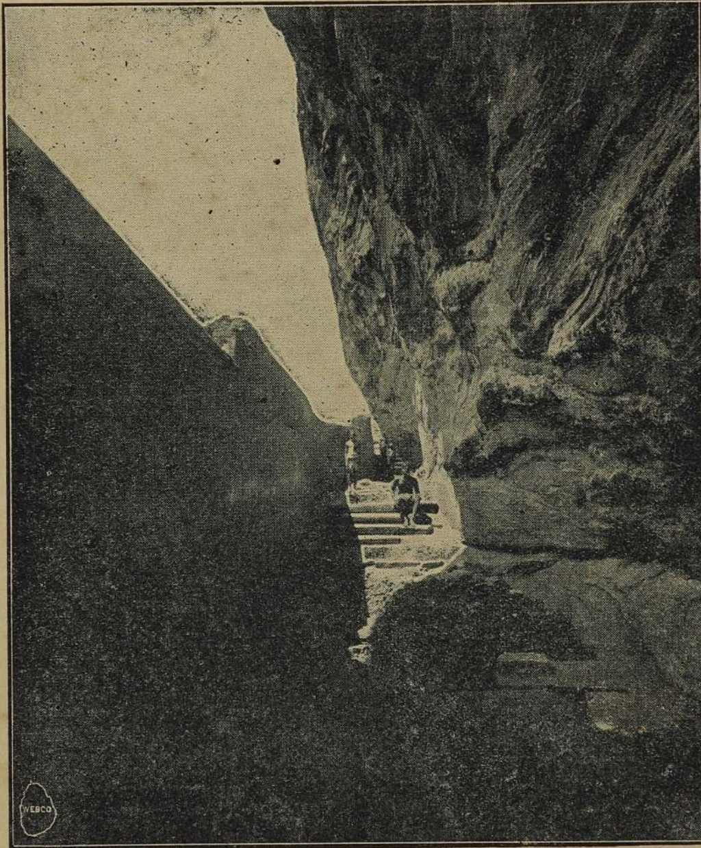
Photograph kindly lent by Messrs. Plate Ltd. SIGIRIYA, CEYLON: THE GALLERY AND THE "CURTAIN" WALL.
