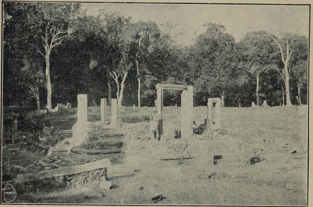
ANURADHAPURA, CEYLON: GEDIGE. BUILDING 'A' UNDER RESTORATION.
