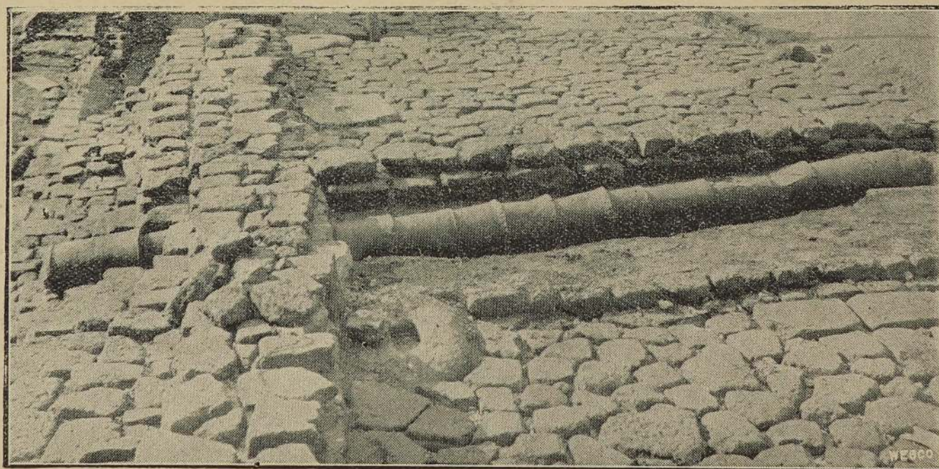
(Reproduced by kind permission of the Archaeological Commissioner, Ceylon.) Polonnaruwa, Ceylon: Terra-Cotta Drain Pipe excavated east of the Palace.
