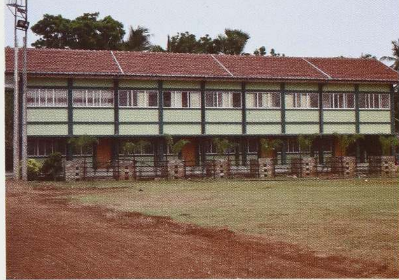
Construction Of Indian Building
