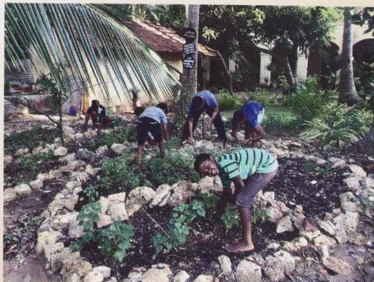
Construction Of Herb Garden
