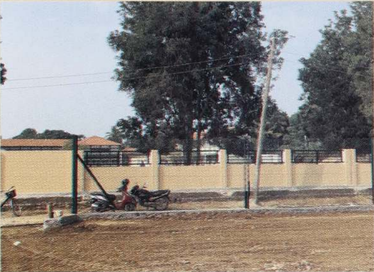
Costuction Of Boundary Wall
