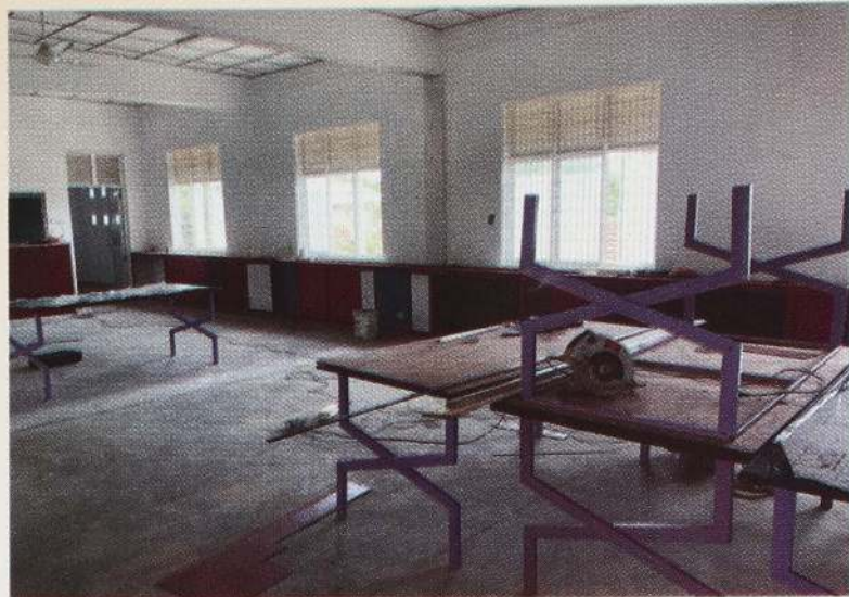
Construction of Science Lab
