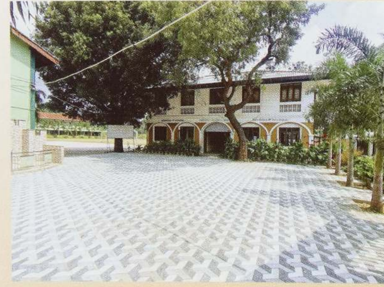
Putting Up Paving Blocks at Entrance Square
