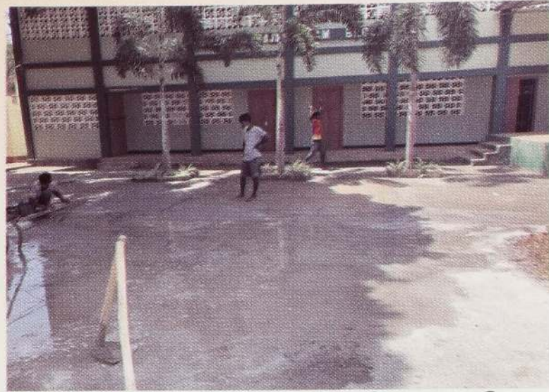
Concrete Floor In front of Rev.Fr.Anton Rajanayagam Block
