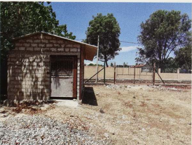
Construction of Store Room for Mini Pitch
