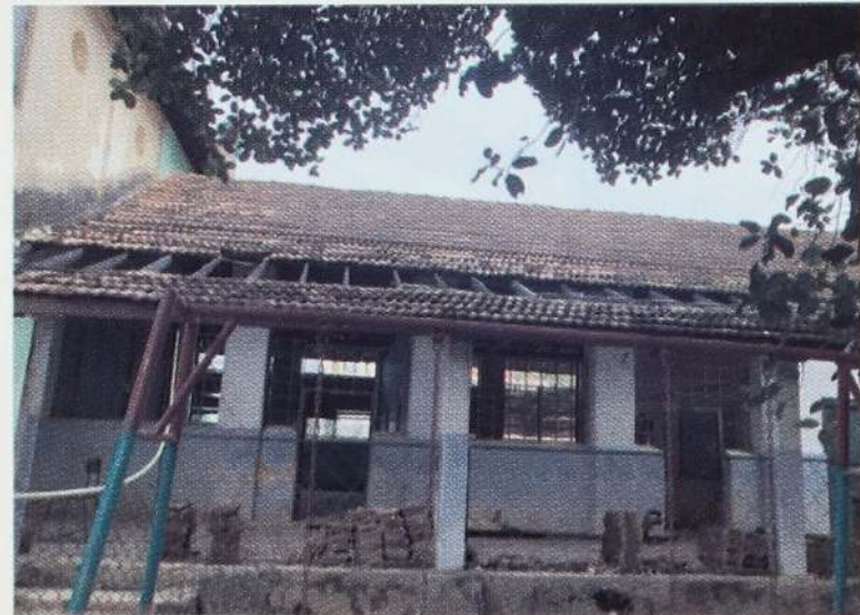
Reparing of Roof
