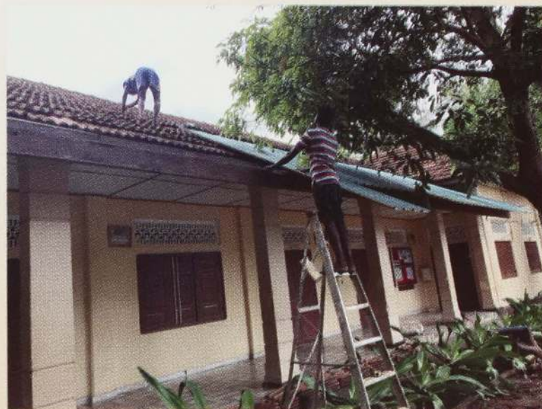
Repairing Of Roof
