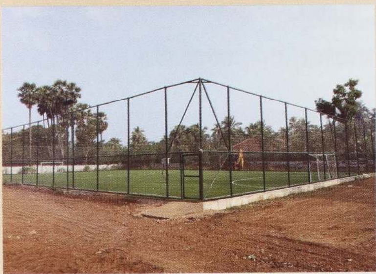
Construction of Internal Fence Of Mini Pitch
