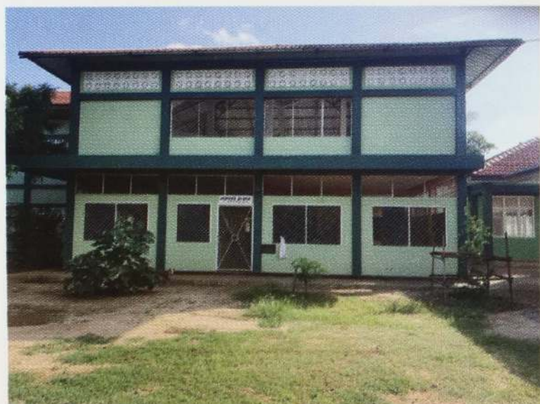
Construction Of Upper Floor of Jeniffer Block
