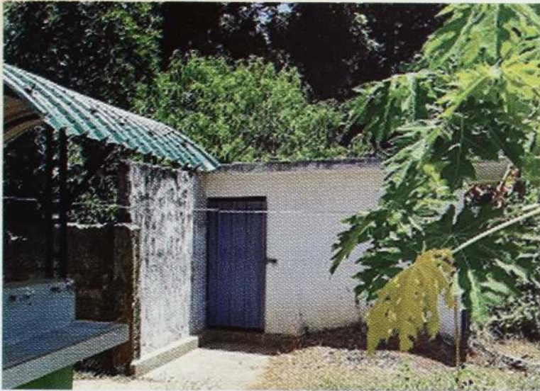
Construction of Wash Room
