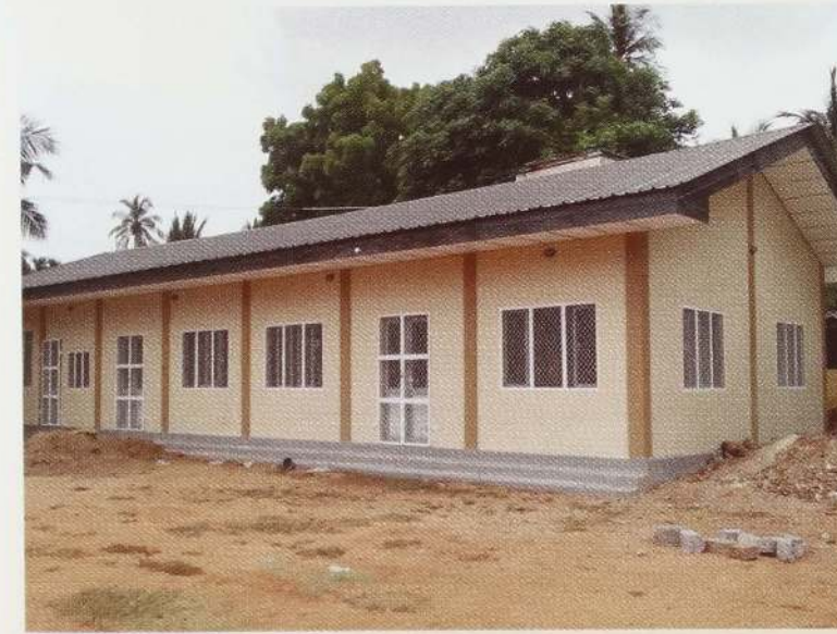
Construction Of Canteen
