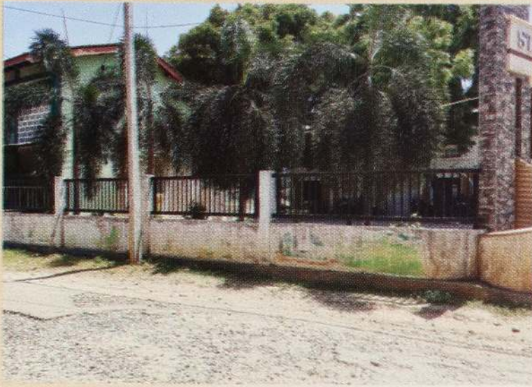
Construction of Boundary Wall
