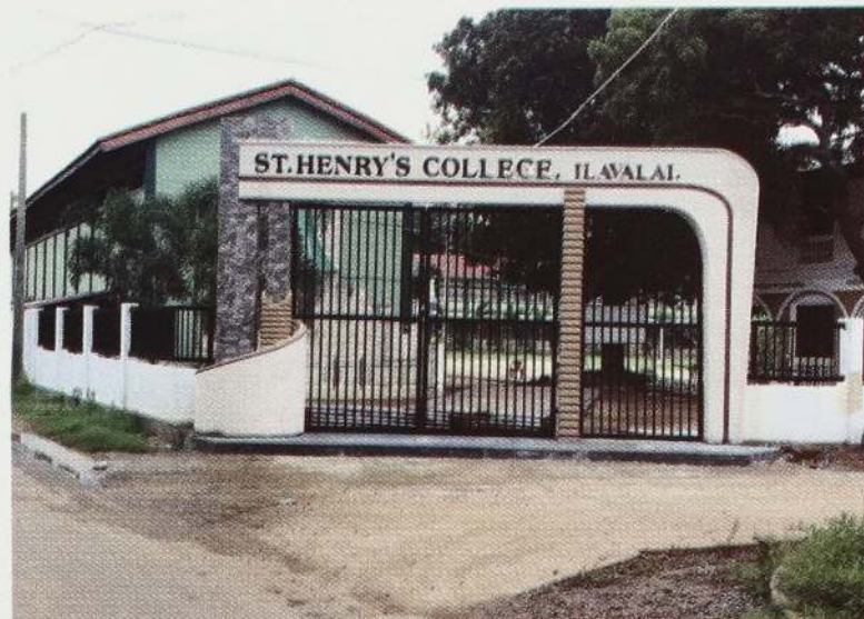
Construction of Entrance
