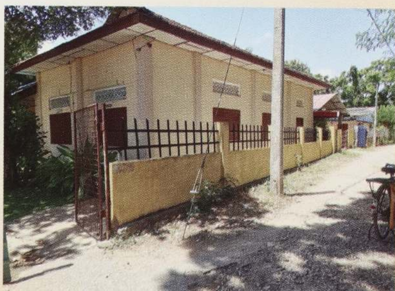
Construction of Bounday Wall
