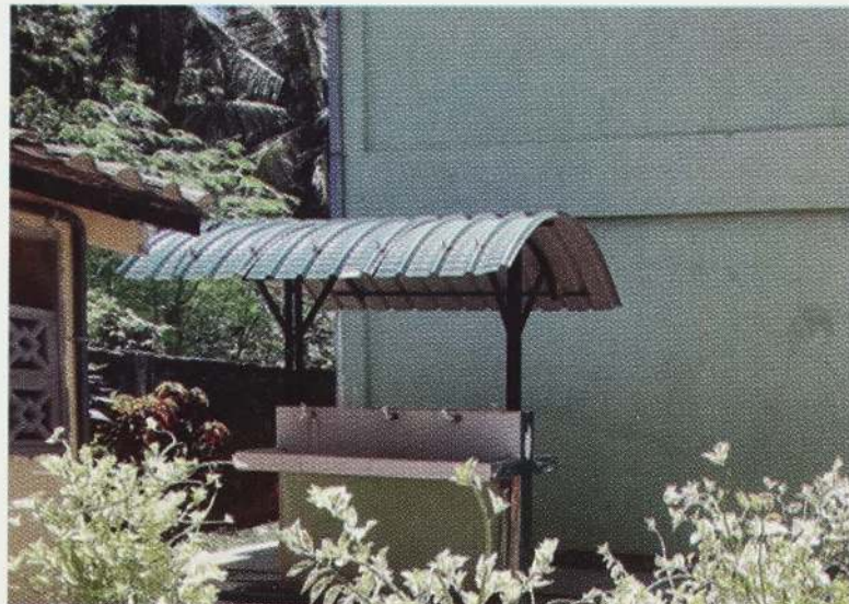
Construction Of Water Taps
