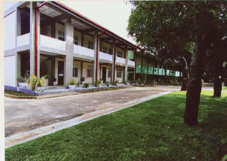
Construction Of Office Building
