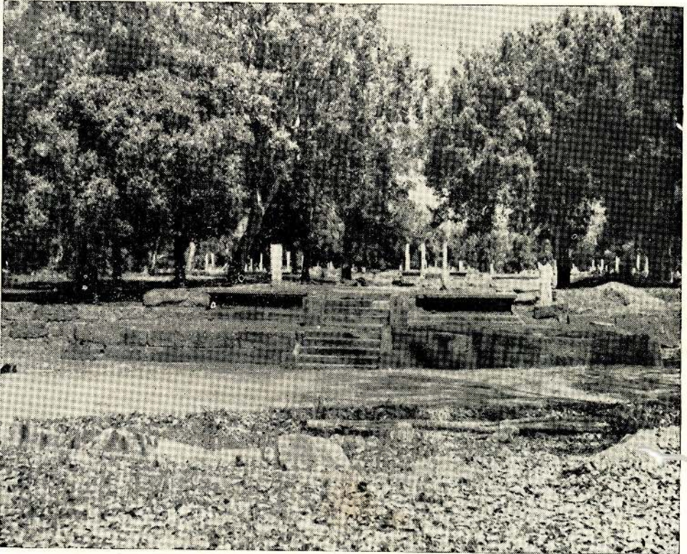
MIHINTALE : KALUDIYA POKUNA, BUILDING ON TERRACE AFTER CONSERVATION
