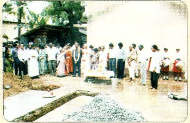
Getting ready to lay the foundation for the 'Hostel Building'
