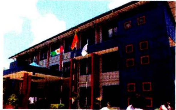
Puttur Sri Somaskanda College – New Building constructed as part of the Mahindodaya 1000 Schools Programme
