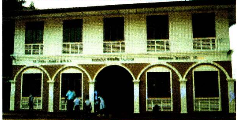
Mankulam MMV School, Thunukkai Zone. New building and computer lab built as part of the '1,000 Schools Programme', also known as the 'Mahindodaya scheme', that is equipping schools with Science, Language, Mathematics, and ICT laboratories
