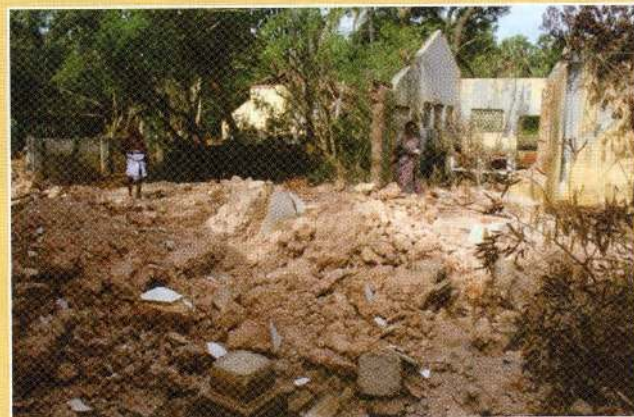
Ayah's house damaged during the war. Picture taken in 2014
