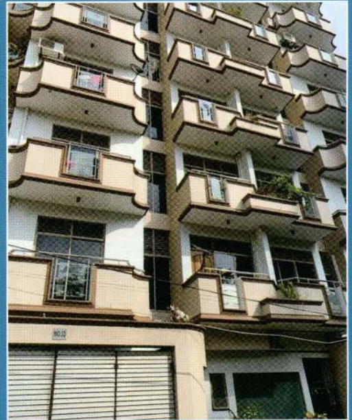
The beloved house the Sangapillai family lived has been demolished and a seven story apartment has come up - 2018
