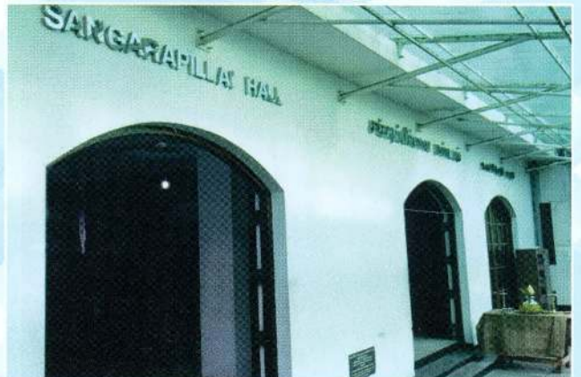
Entrance of the Sangarapillai hall
