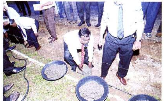
laying foundation stone for the New Library Building 2017
