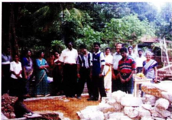
Laying of foundation stone for new workshop on 2003/02/12 in our premises
