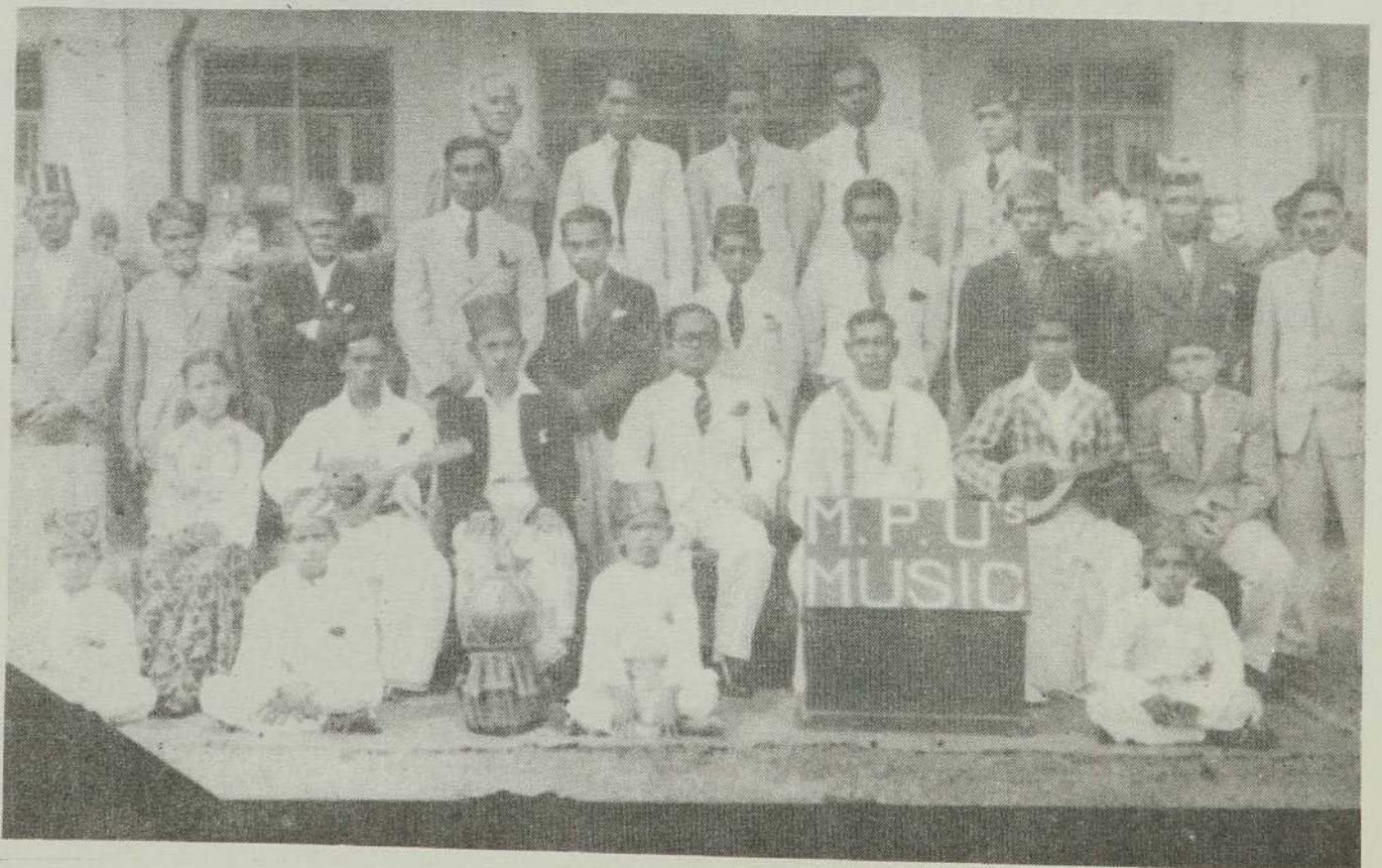
Malay Progressive Union Members - 1936 Seated in the centre Dr. M.P. Drahman Member of Parliament 1956-1960
