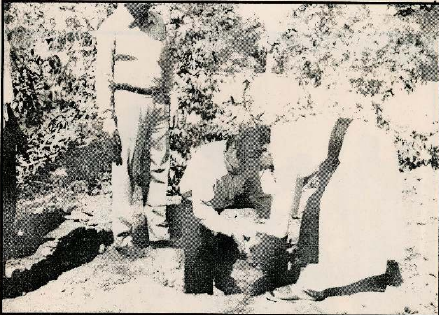
Laying of Foundation Stone to the College Church
