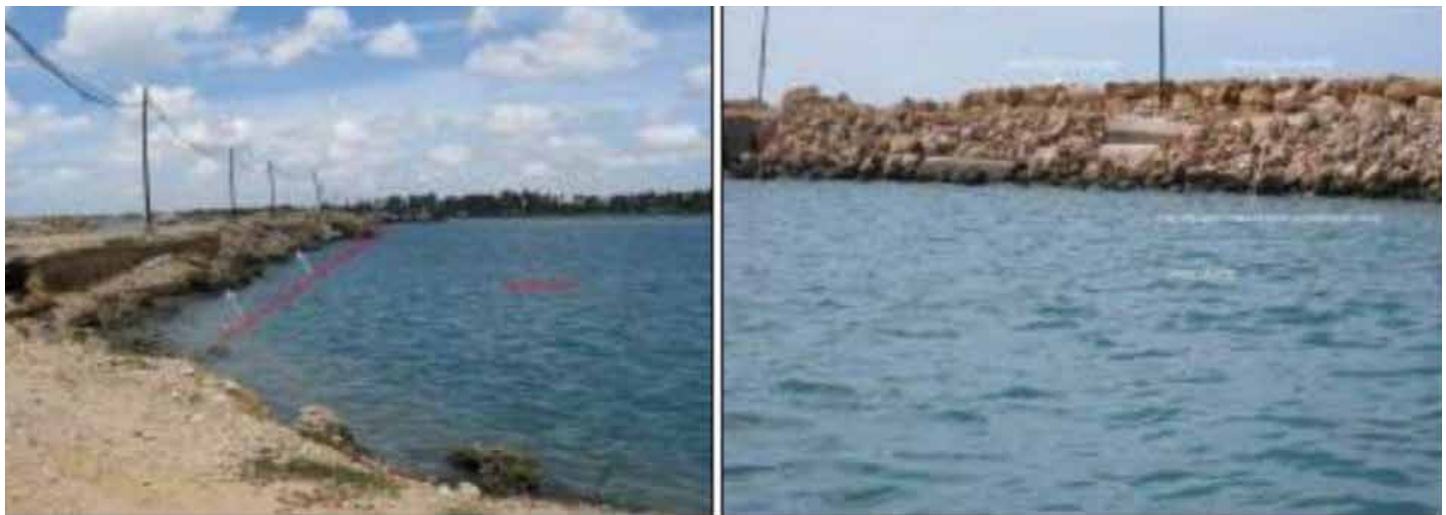
Figure 2.4: Condition of the Existing Breakwater
