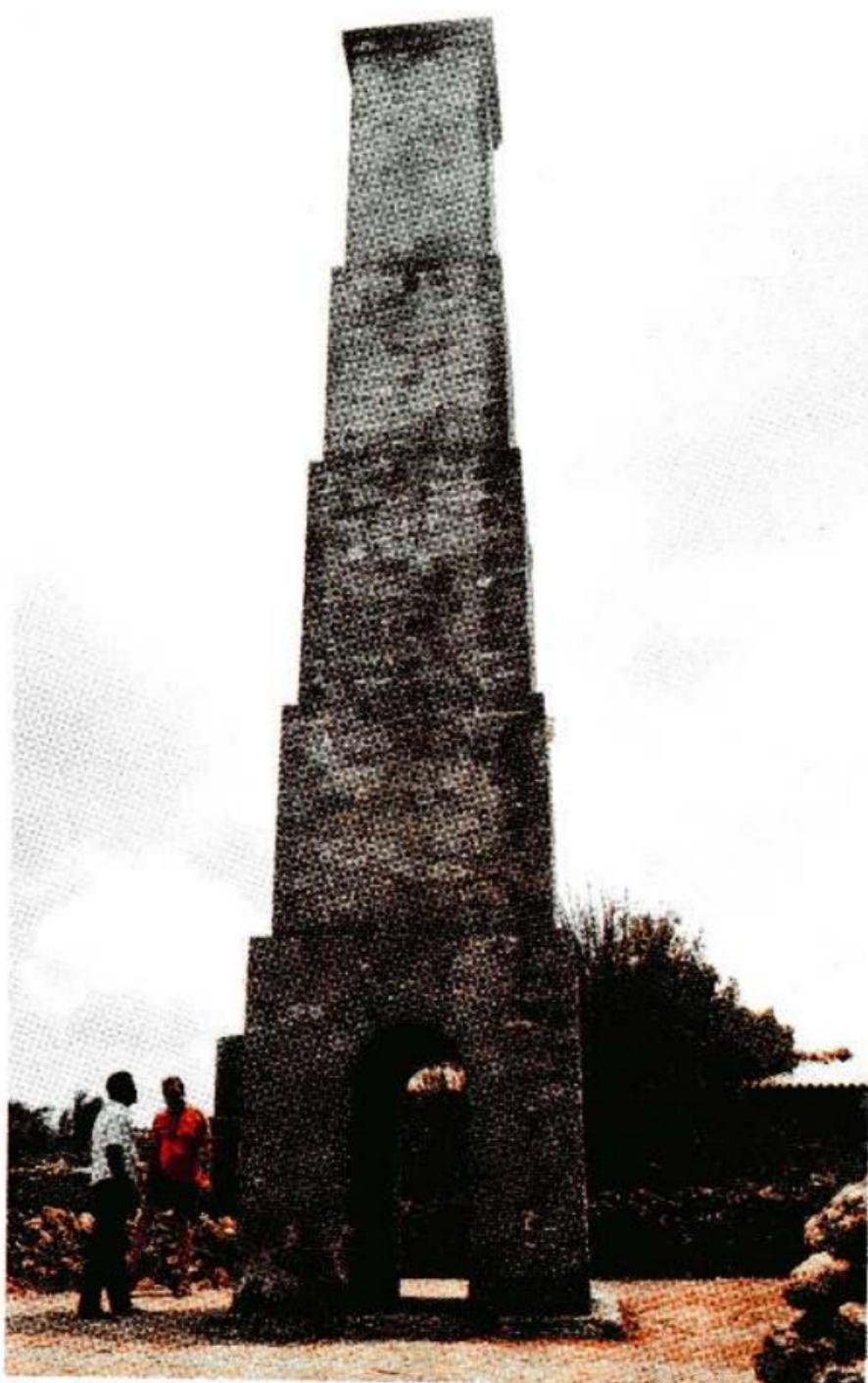
It is a light house built by Dutch using coral stones. It was the practice to set fire on the basement and its sparks travel through a small tunnel upwards. The light seen on the top of the lighthouse indicated the location to sailors or fishermen in the night. In 1905 it was reconstructed by British. It is located in the south of Delft.
