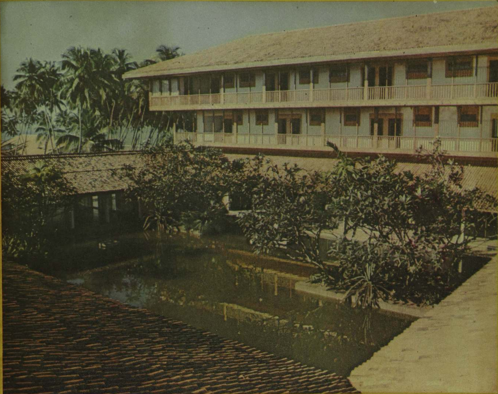
AN ATTRACTIVE RESORT COMPLEX HAS BEEN DEVELOPED ON THE SOUTH WEST COAST
