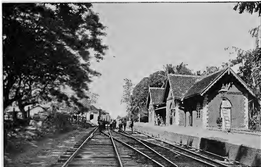
93. HENARATGODA RAILWAY STATION.
