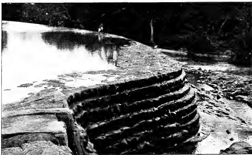
177 ANCIENT SPILL BY WHICH THE OVERFLOW OF A RIVER IS DIVERTED TO THE GIANT'S TANK. (Photograph by Owen W. Herman, Esq.)
