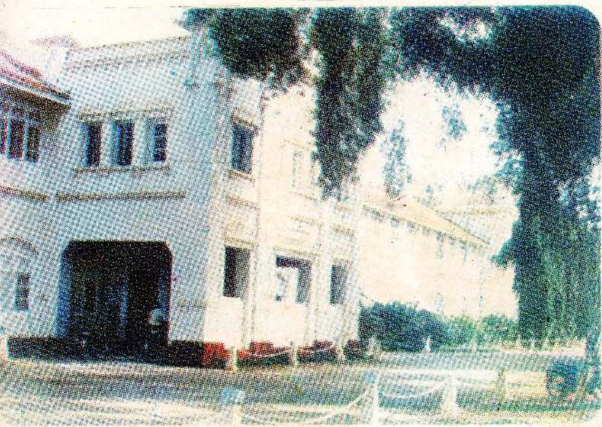
Front View of the Ramanathan Block after renovation.
