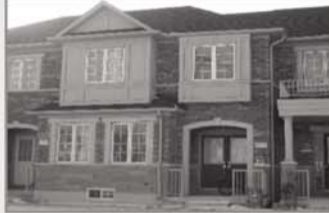
14th Ave/Box Grove By-pass
