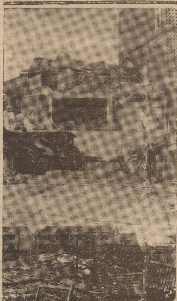
Top: Bazaar Area Centre: K.K.S Road near the Jaffna Fort Bottom: Damaged Telecommunication Centre
