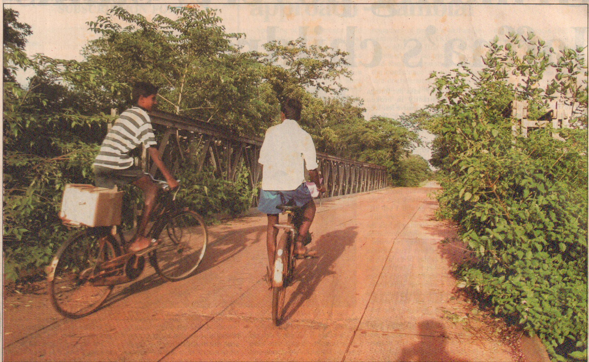
Boy on bicycles pedal across a brand new bridge built by the Sri Lanka army at Olumadu, east of Mankulam after fighting in Operation Jayasikurui destroyed the original bridge
