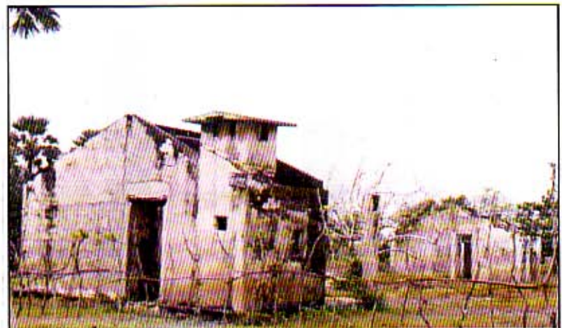
Pinaimurunkayadi Housing Scheme –Navatkuli
