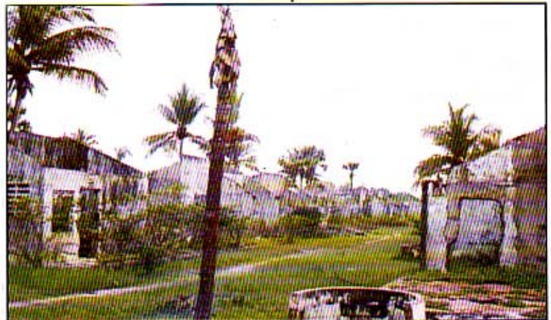
Pommaiveli Housing Scheme
