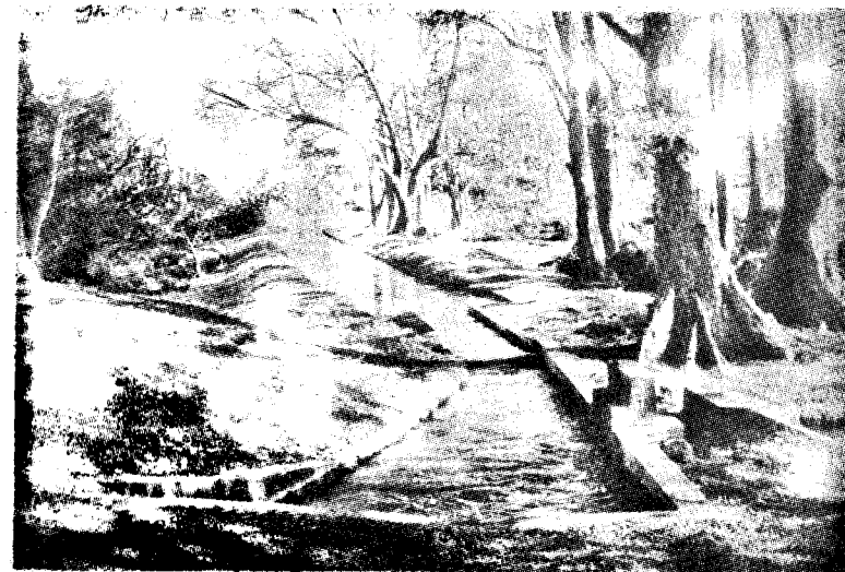
18.8 HINGURA ARA TANK D/S OF SLUICE & CHANNEL
