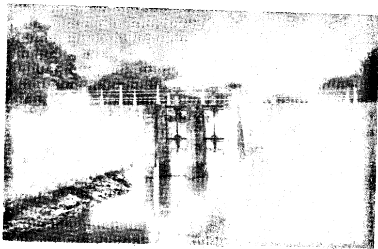
18.1 UGGALKALTOTA L.B. CHANNEL HEAD SLUICE
