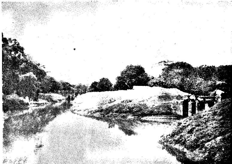
90.14.4 AKKATHIMURIPU INLET CHANNEL & SLUICE
