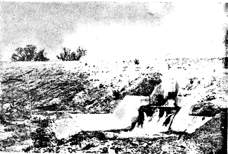
60.36 KAUDULLA TANK—D/S OF SLUICE
