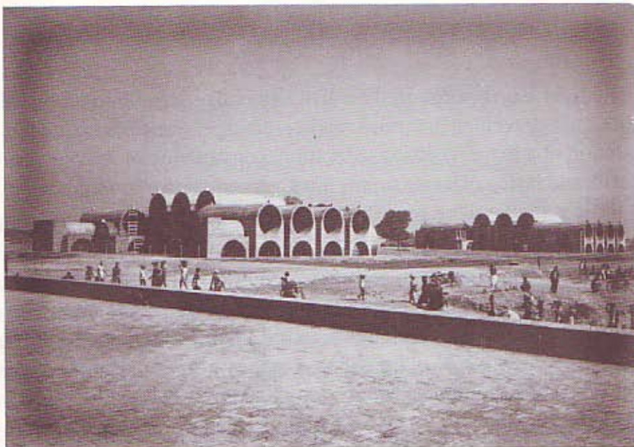
Museum, Library & Central Link bridge
