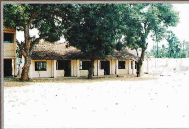
3 class rooms in the western side with closure doors and windows supported by the Foundation
