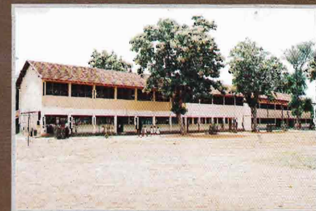
Eastern side view of the college in front children are playing. First story is supported by the Foundation
