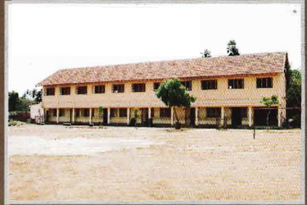
Up stair of the building partly finished is now completed and painted with the support of the Foundation
