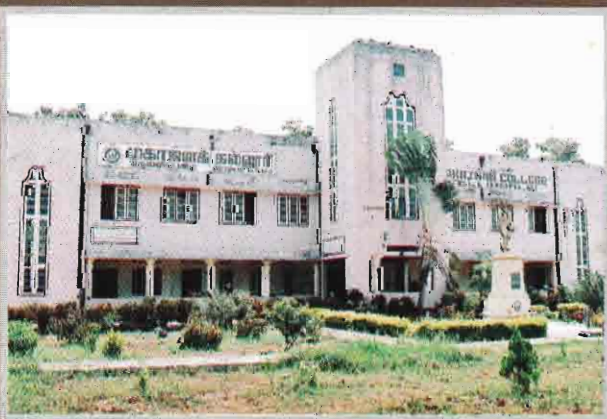
The Main Thuriappah building, work to renovate the building and full painting work commenced and in progress.
