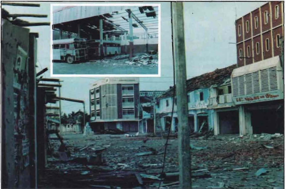
Jaffna Town Centre and Bus Station devastated by the Sri Lankan military
