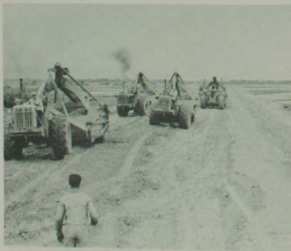
Road construction in Laos with American equipment.
