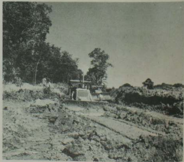
Construction of Serian-Simanggang Road, Sarawak.
