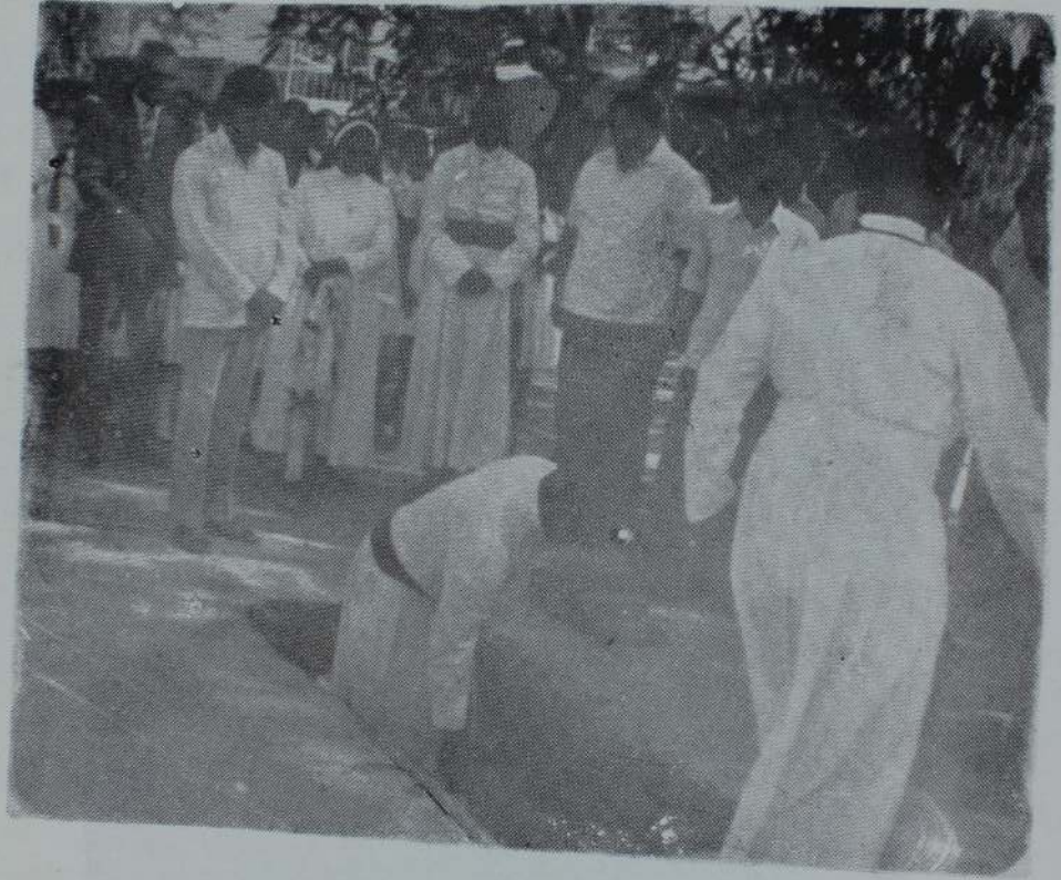
Laying of the foundation stone for the Advanced level Science Laboratory 1986.
