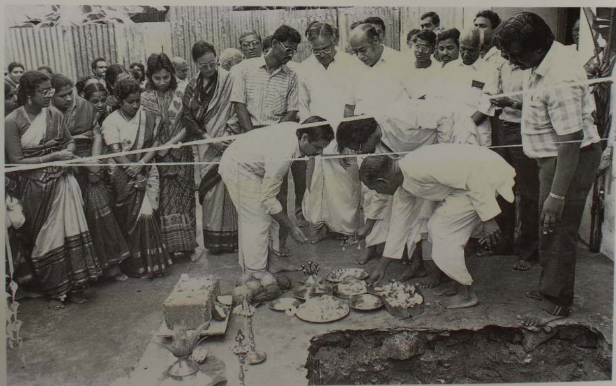
'MANIAN' GETTING READY TO LAY THE FOUNDATION - 6/5/1990
