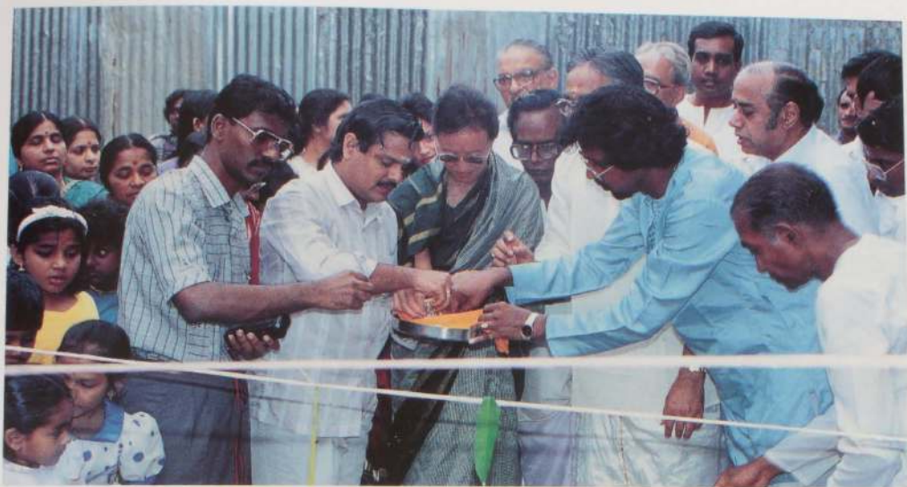
GETTING READY TO LAY THE FOUNDATION ON 6TH MAY 1990
