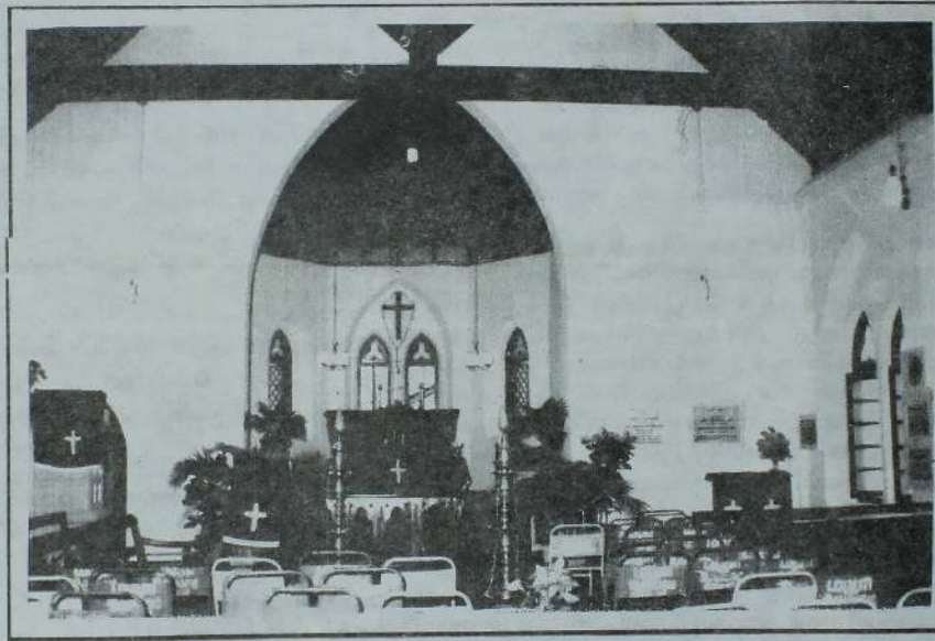
CHANKANAI - CSI Church Renovated and Rededicated on 13th July 2001
