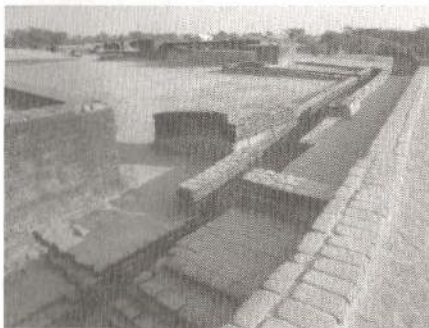
Acropolis with drains
