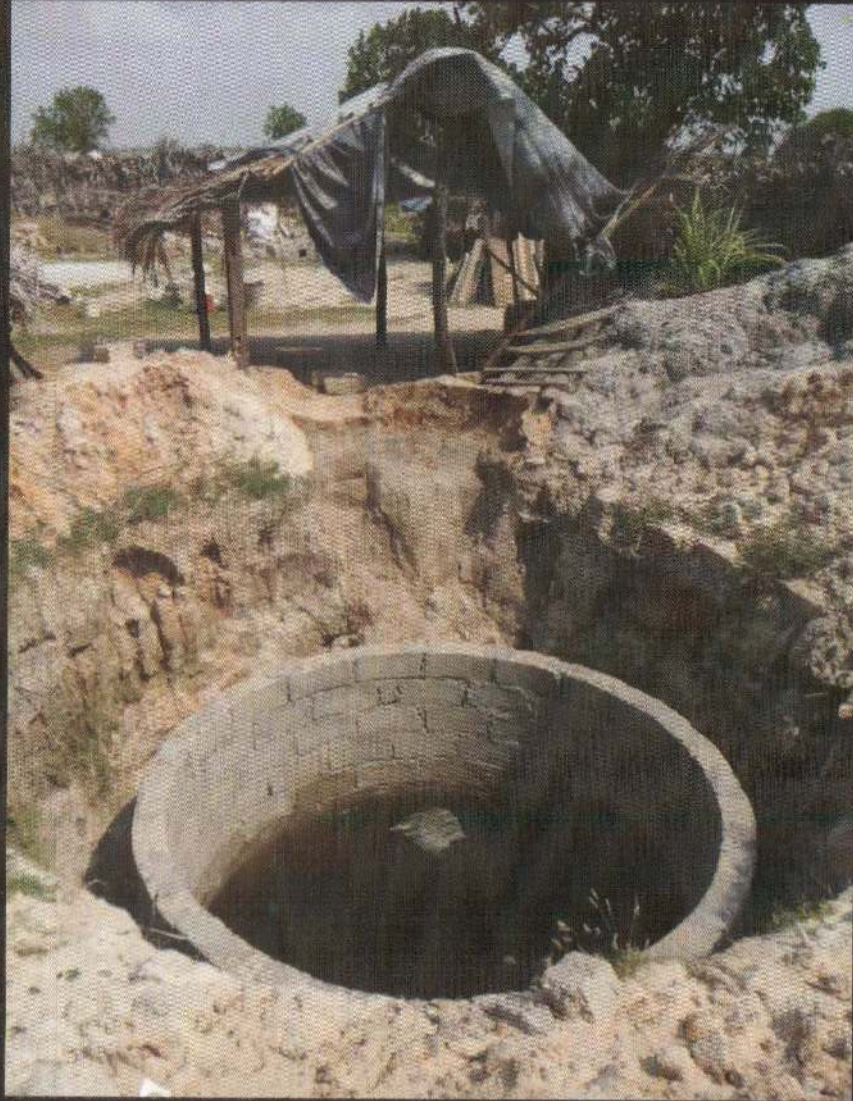
A well in construction
