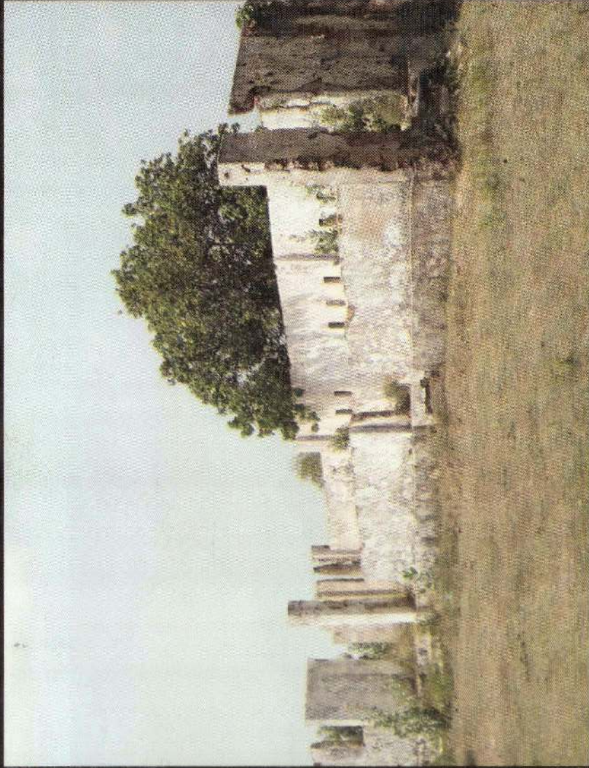
A damaged house
