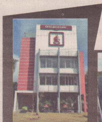
Nellyady Branch Building
