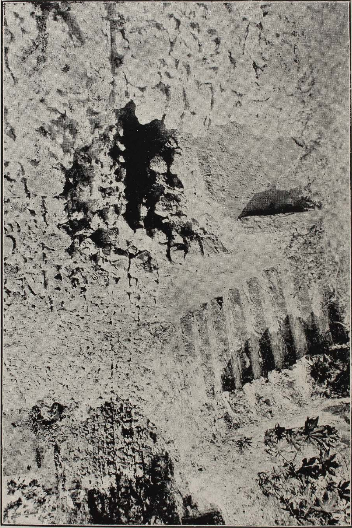
PLATE IX.—DELFT FORT.—Ruins from the north-east. Showing remnants of staircase A and entrance to room 4. (Note the coral of which the fort was built).
