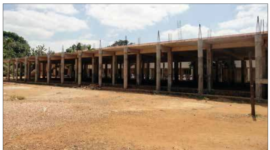
Sanders hall under construction
