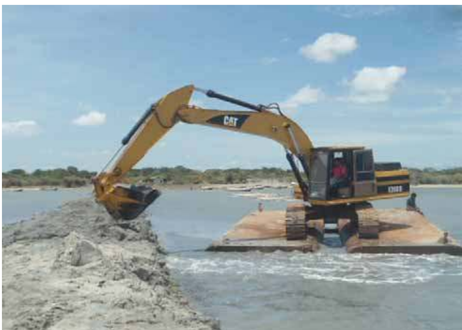
A back hoe at work in one of the sites
