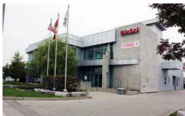
Building Front View
