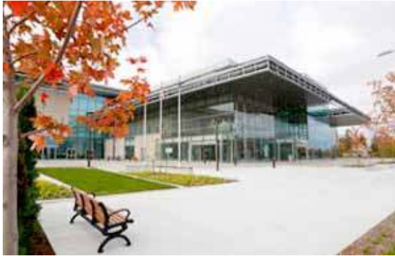
Pan Am Centre Exterior
