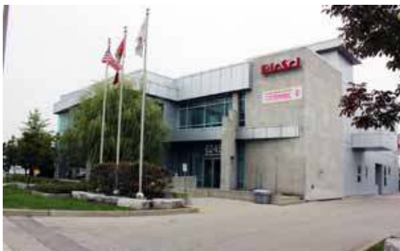
Building Front View
