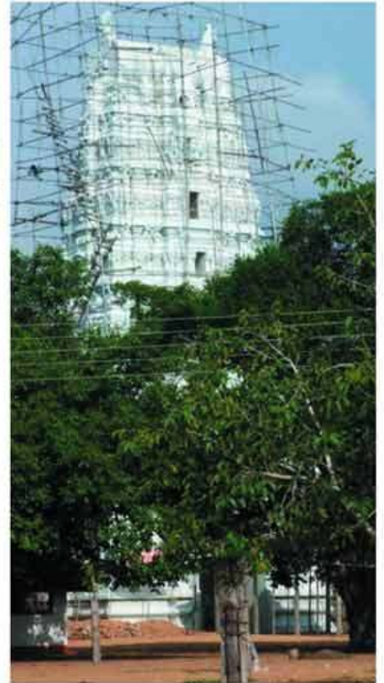
Kopuram under construction
