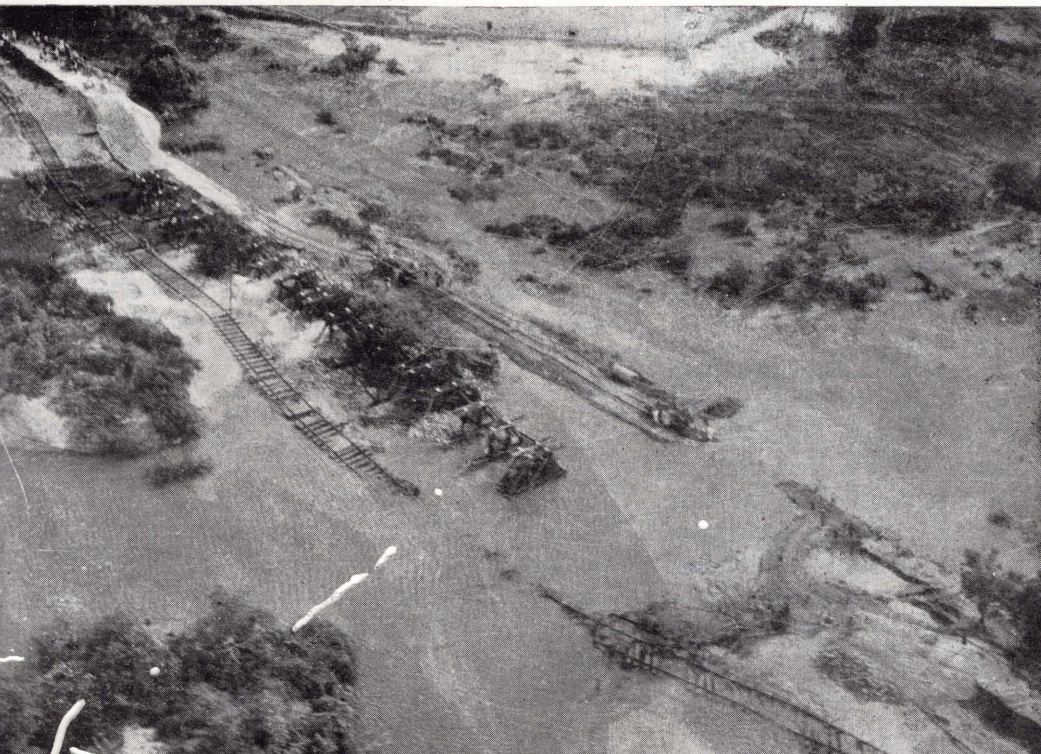
Road and railway track washed off by floods in the Eastern Province
