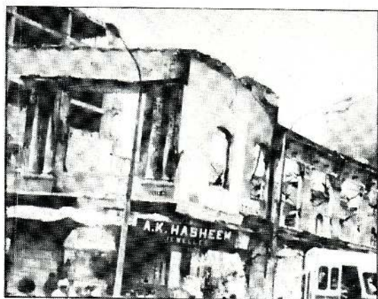
A ravaged building (the former Bristol Hotel) in Fort.
